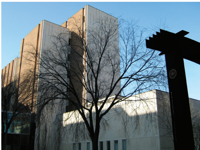
University of Alberta, Chemical and Materials Building
