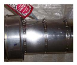
STEP 5: Insert the exterior sell inside the outer wall of the Secure Seal part and tighten the screw. Install the outer collar and tighten to finish installation
