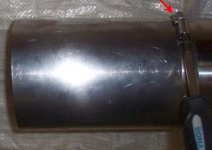
STEP 3: Place the two remaining inner collar over the inner wall and insert the male end of a Secure Seal part inside the inner collar. Make sure the inner wall is well positioned over the O-ring before tightening the collar. Position the draw band and tighten the three collars firmly.
